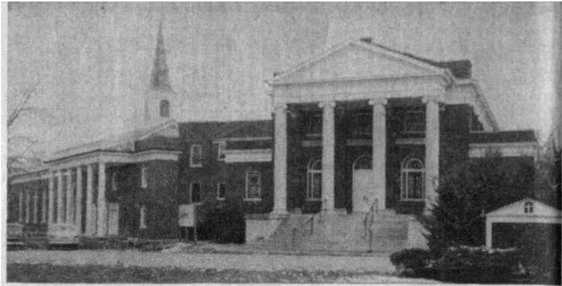
A new sanctuary (left) of Colonial architecture was added to Beargrass Christian Church. The old Grecian columns (right) were torn down. (See photo page one).
