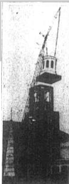
Rather than build the steeple in the air, the contractors, Otto Tapp & Sons, built it on the ground and then hoisted it (left) into place atop the beautiful new sanctuary at Broadway Baptist Church. The steeple is 126 feet tall. The new sanctuary (right) is rapidly approaching completion, and in size dwarfs the present sanctuary, a portion of which is visible at right. These photos were taken on Monday.
